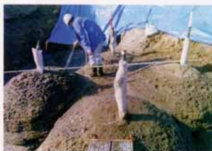
Improvement in Progress (Field Positive Test)
