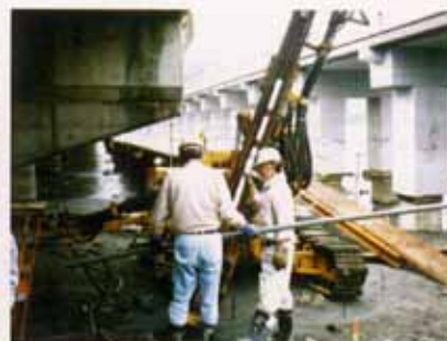
Feeding Pipe Pitching
